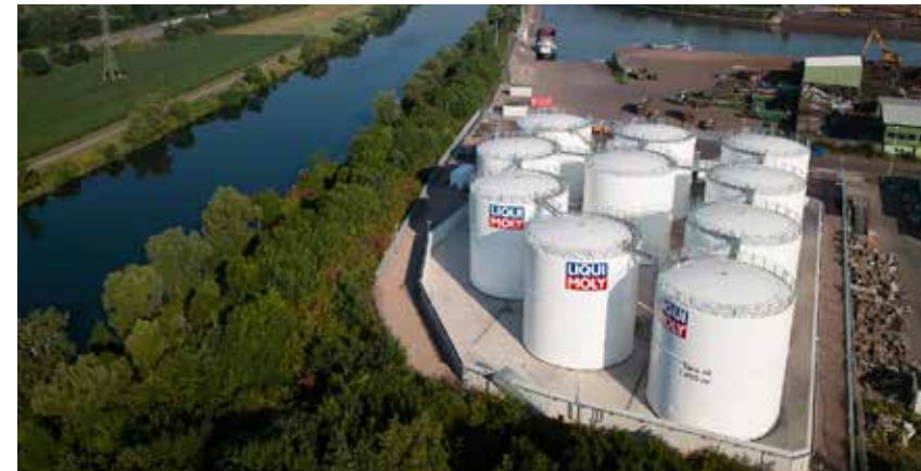
The LIQUI MOLY tank farm in Saarlouis, Germany.
